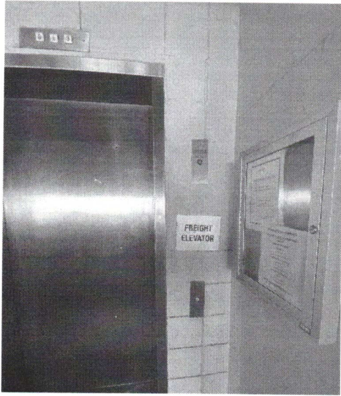
25. South – New vandal-resistant corridor fixtures are recommended.
