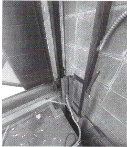
38. North – New car positioning device to be installed.
