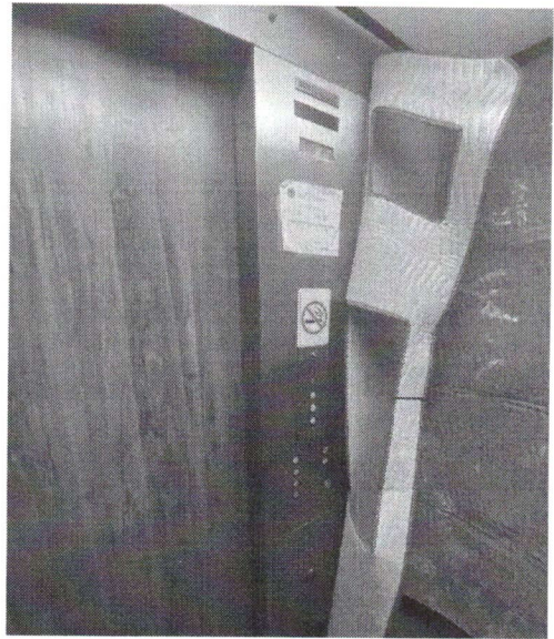
26. South – A new car operating panel with vandal-resistant buttons and operational switches and signals to be provided.
