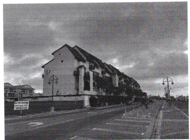
Figure 2: View of the south elevation.
