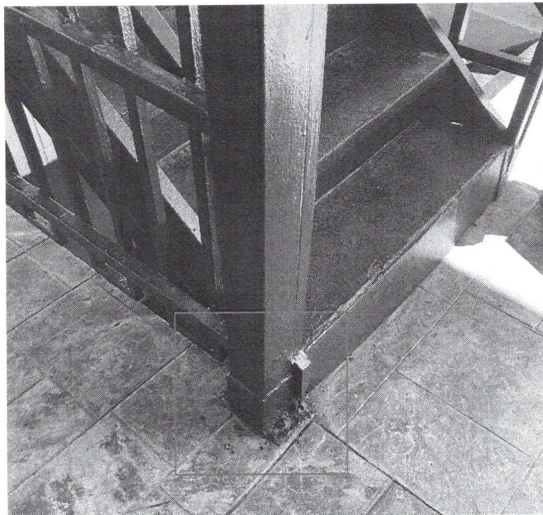
Photo No. 17 – West Stairwell Type I Repair
