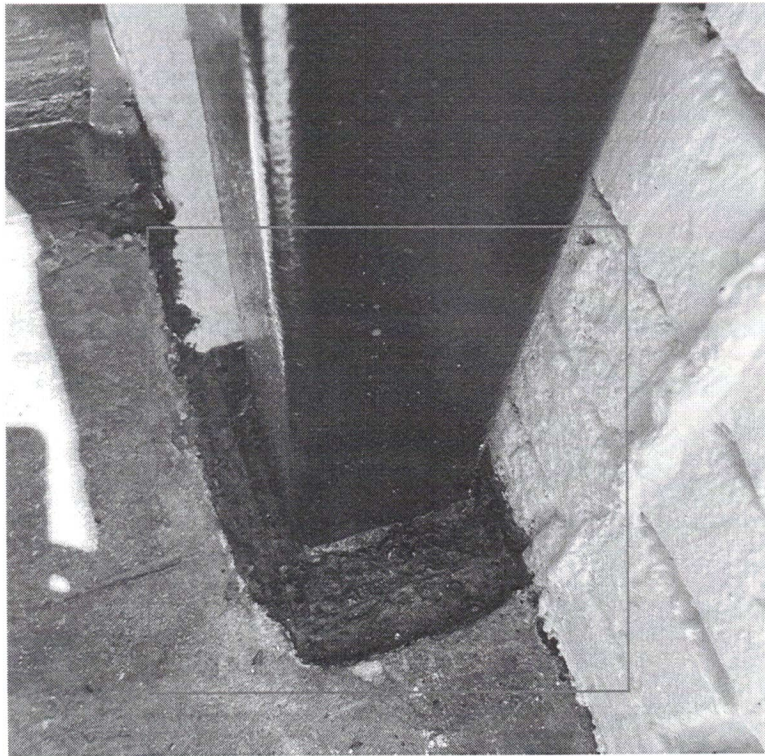
Photo No. 18 – West Stairwell Type I Repair
