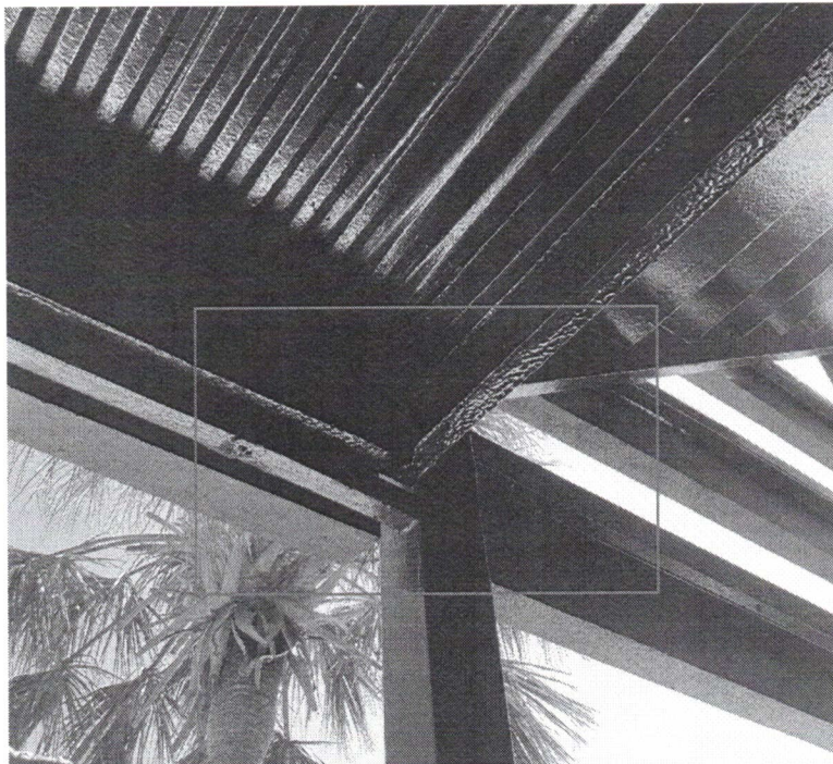
Photo No. 19 – West Stairwell Type I Repair
