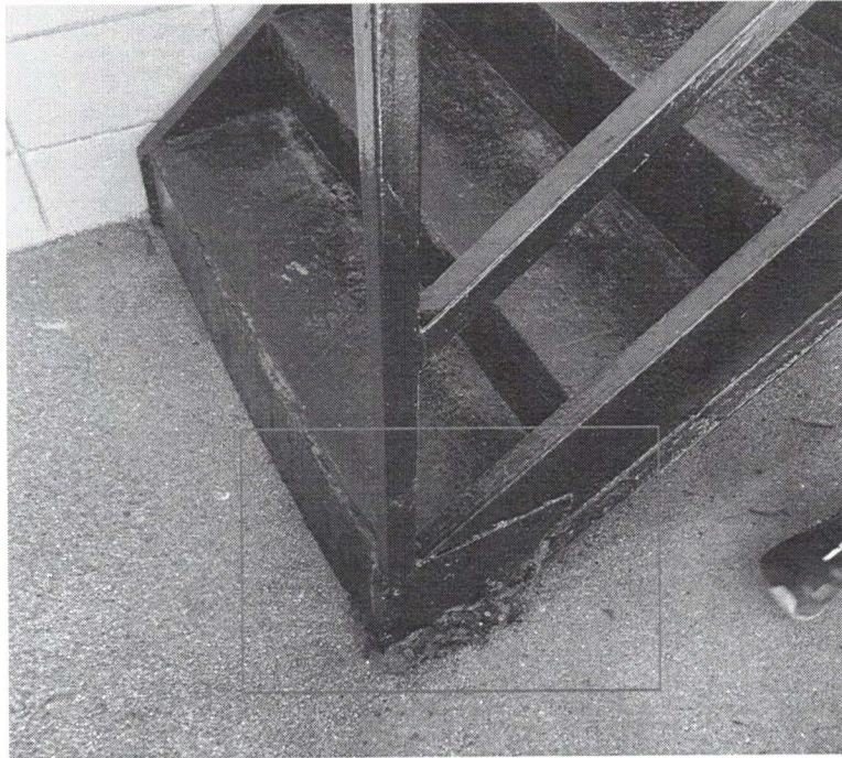
Photo No. 22 – West Stairwell Type II Repair
