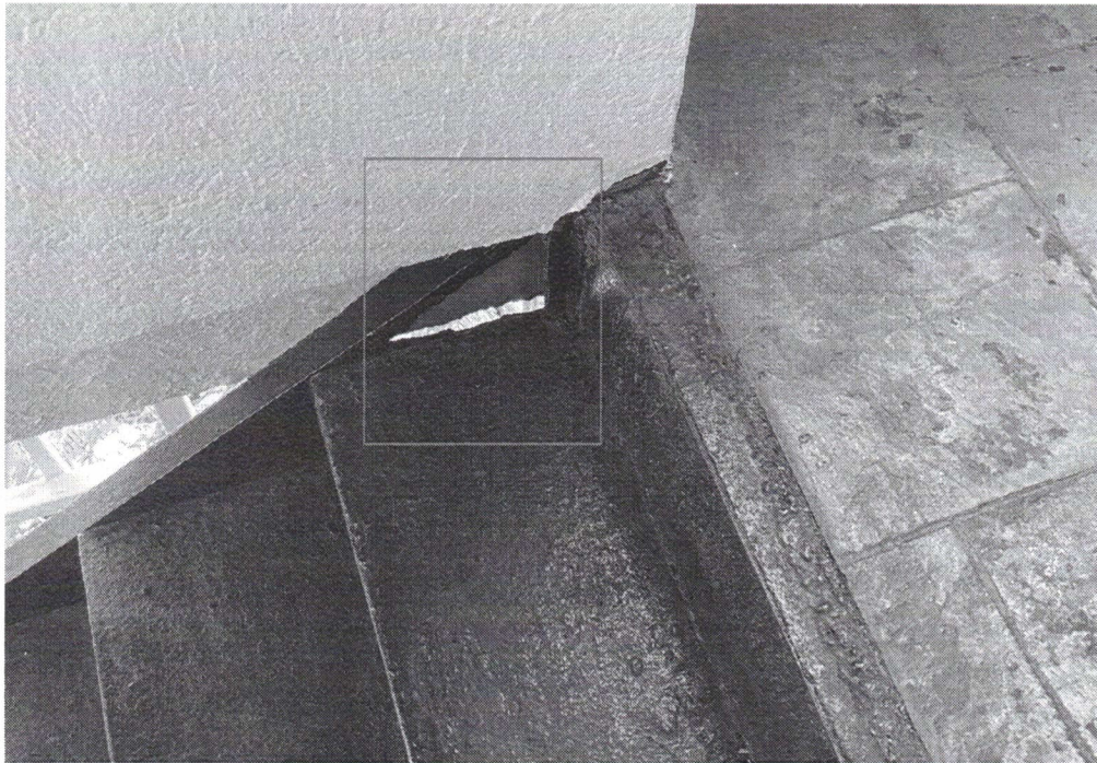
Photo No. 11 – Center Stairwell Type II Repair
