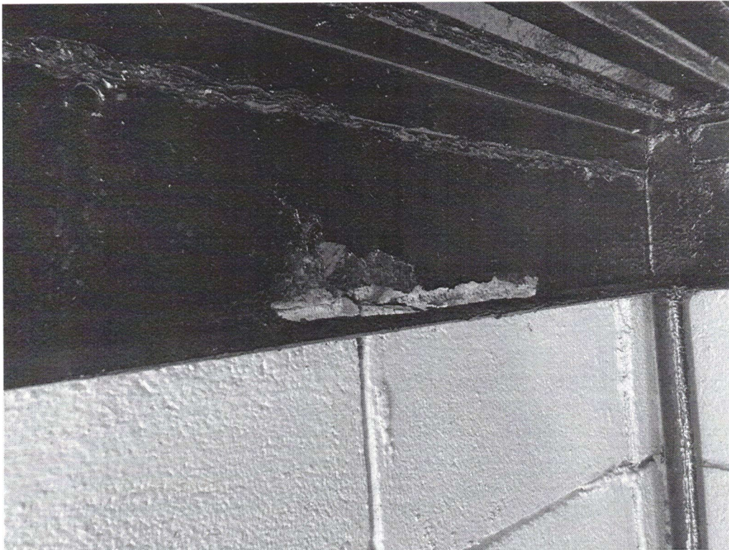
Photo No. 7 – South Stairwell Type II Repair
