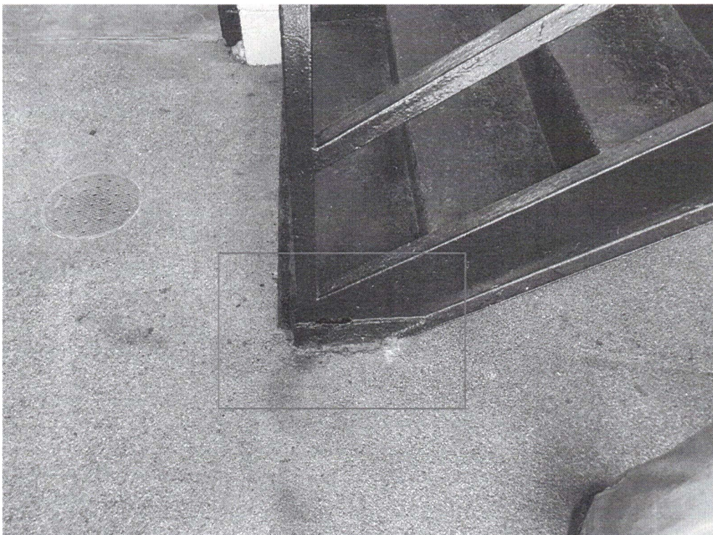
Photo No. 13 – Center Stairwell Type II Repair
