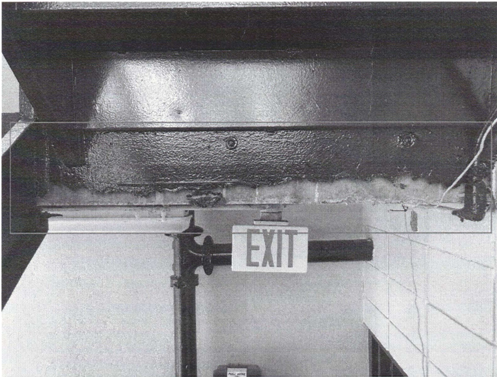
Photo No. 12 – Center Stairwell Type II Repair
