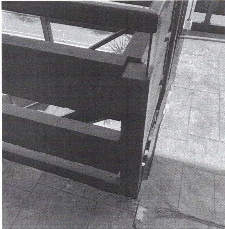
Photo No. 15 – West Stairwell Column Repair Location No. 4
