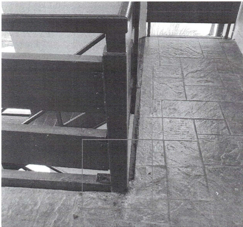
Photo No. 8 – Center Stairwell Column Repair Relocation No. 3
