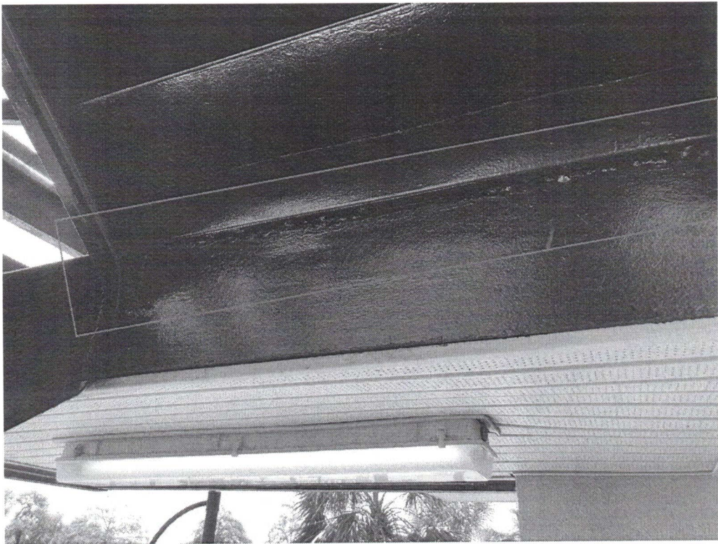
Photo No. 16 – West Stairwell Type I Repair
